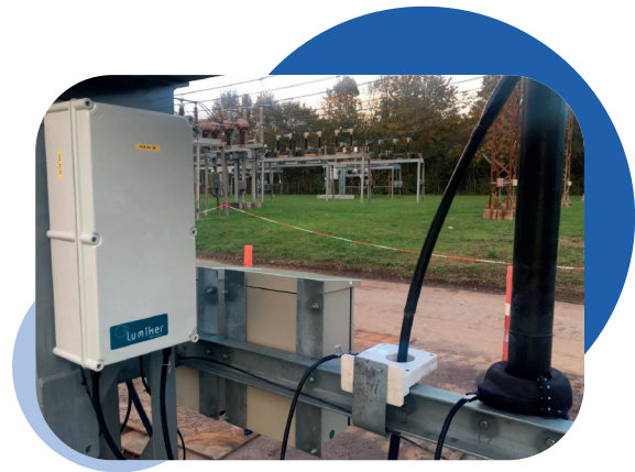
Seath OCT, HV cable OCT and multiplexer
