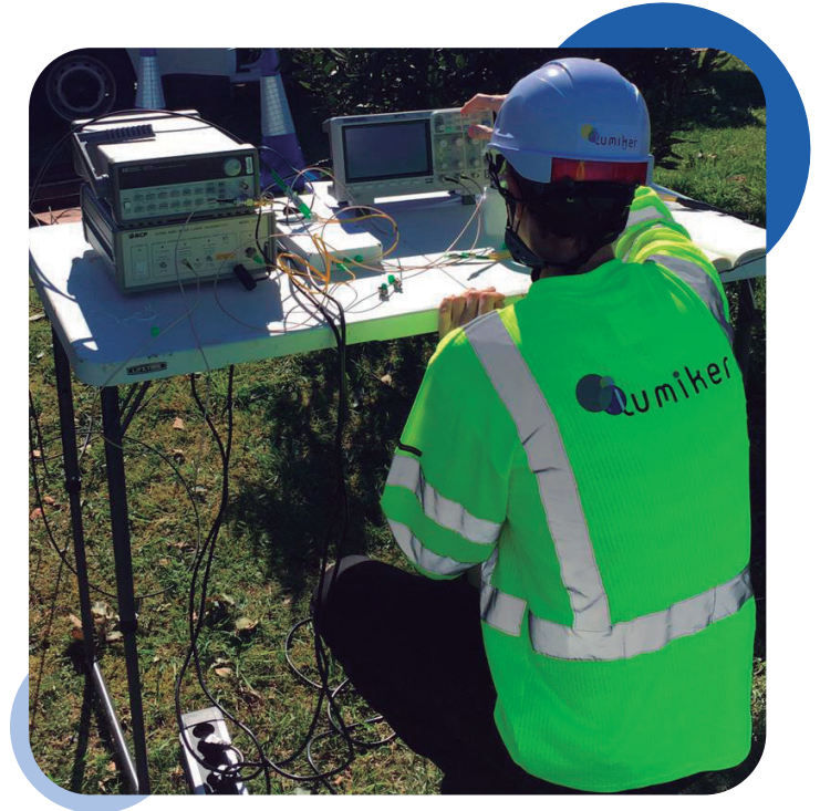
STS Installation tests
